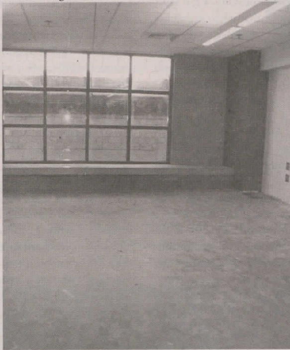
The unfinished lounge area
